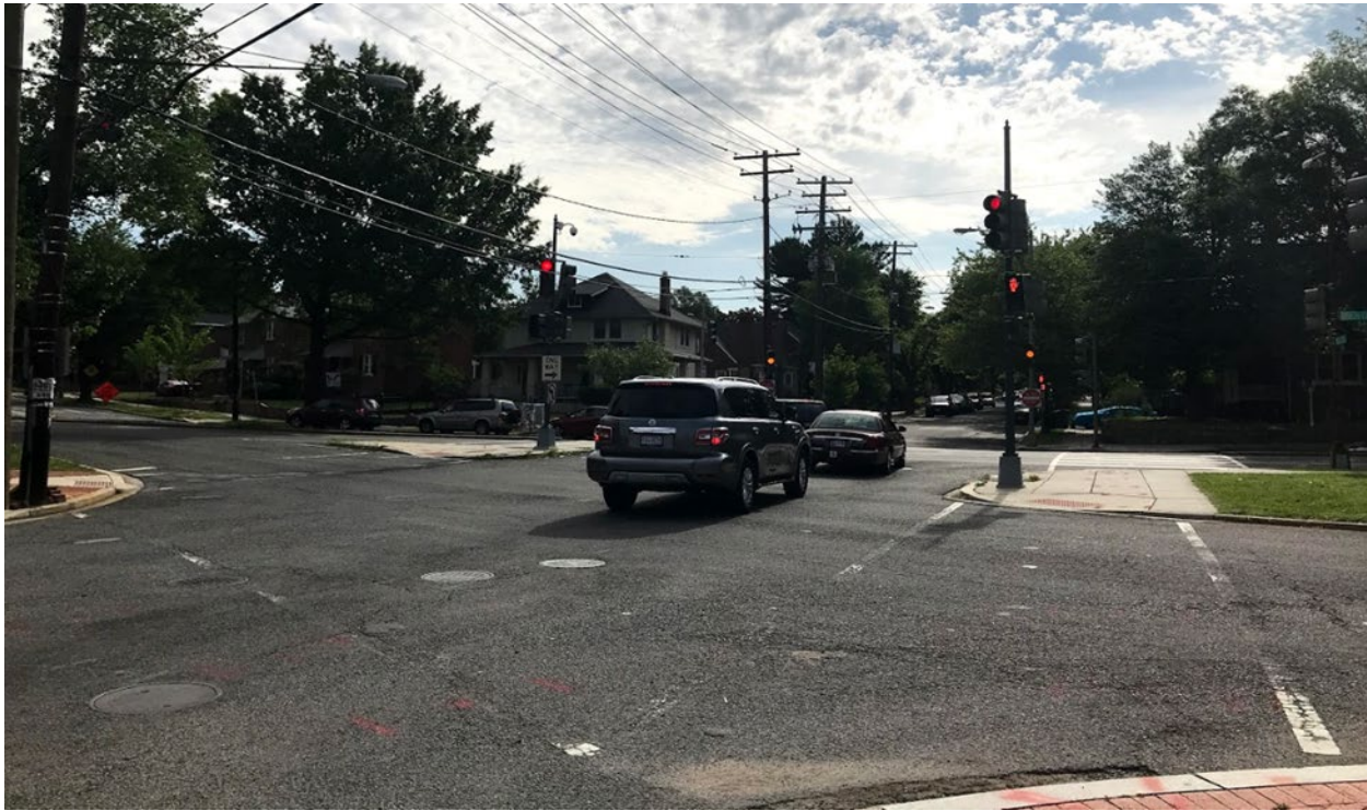
Figure 1: Crosswalks on New Hampshire Ave and Kennedy St are in poor condition
