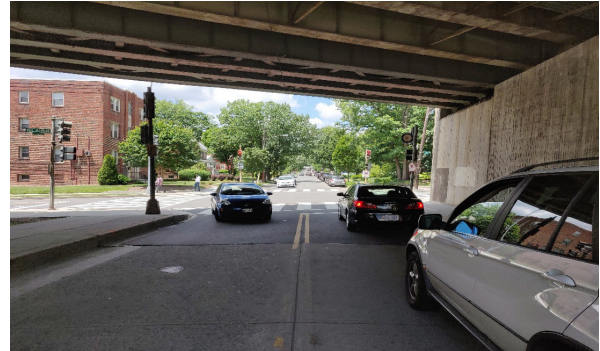
Westbound Approach on Aspen Street, NW with double yellow centerline marking
