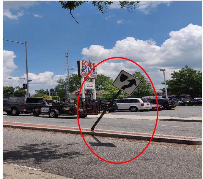
Bent signage on Alaska Avenue, NW
