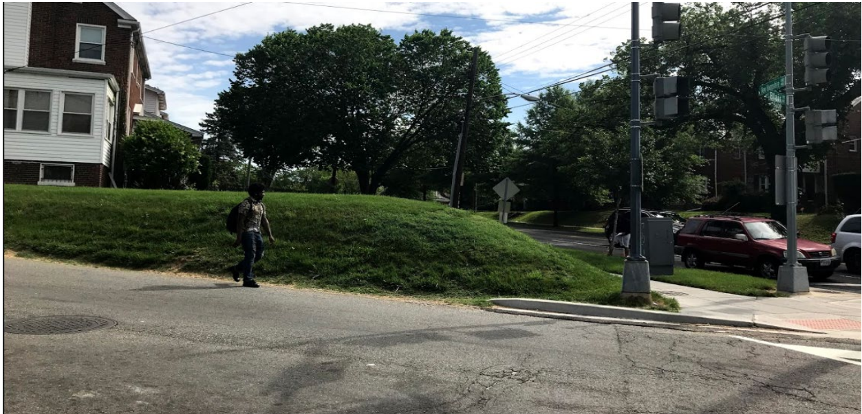
Figure 2: Missing sidewalk Due to Existing Topography along Blair Road NE
