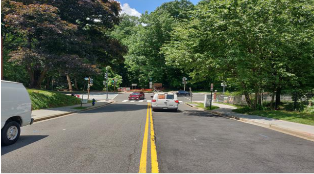
Westbound Approach on Aspen Street, NW with double yellow centerline marking
