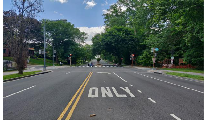
Southbound approach on 16 th Street, NW with double yellow centerline marking and exclusive left turn (only) lane
