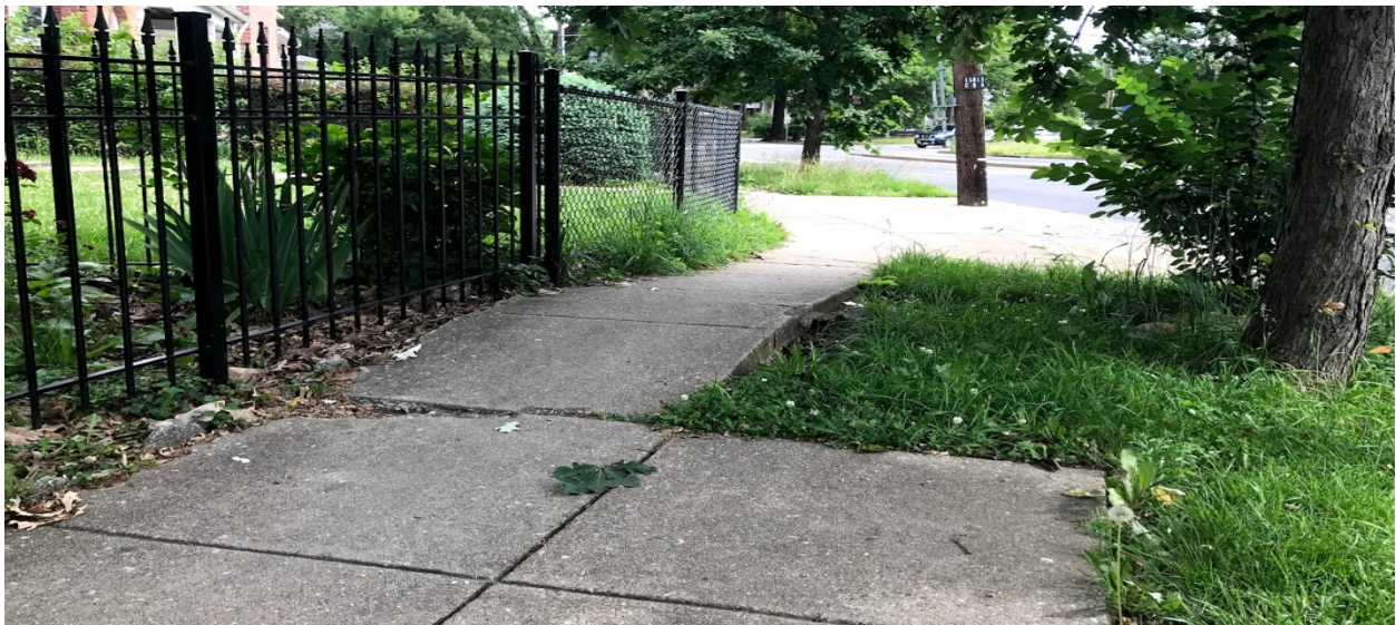
Figure 3: Sidewalks along New Hampshire Avenue
