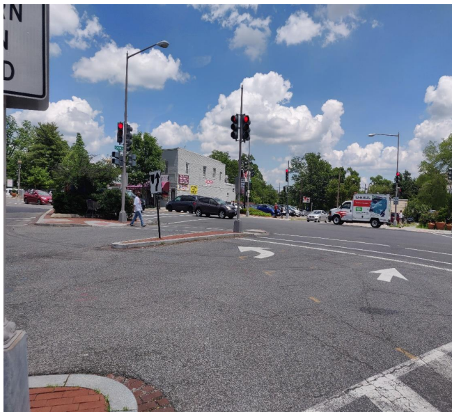
Signal heads and Street lights at intersection
