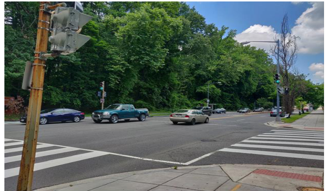
Signal heads and street lights at intersection
